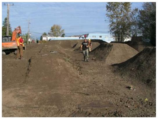
Once the park was this far, capping material brought in by the city was installed for better drainage and five more days of detailed lip, transition and drainage shaping all compiled to create all weather riding potential.
