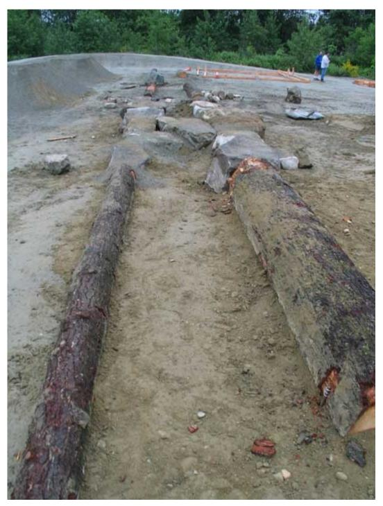
The skills park was to be a all weather park so it was built with sand clay base and then capped with a screening material similar to materials Hoots had used in West Vancouver and Richmond. One of the side advantages to bringing in the materials was that it kept crews from passing through capping material when digging material out for footings as well as knowing what the final product was going to look like.
